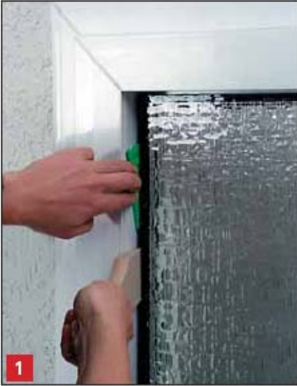
Figures 1 & 2: Insertion of the packers on the closing side
